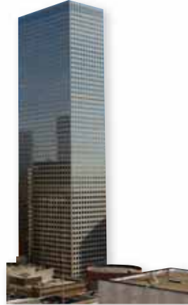
Seagram Building New York, NY 38 Stories: 515 ft 820,000 ft 2 floor space
