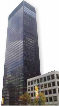
Republic Plaza Denver, CO 56 Stories: 714 ft 1,340,000 ft 2 floor space
