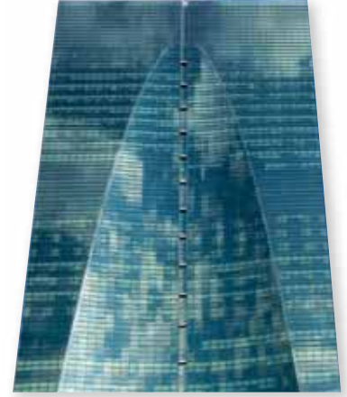
Espirito Santo Plaza Miami, FL 37 Stories: 483 ft 750,000 ft 2 floor space
